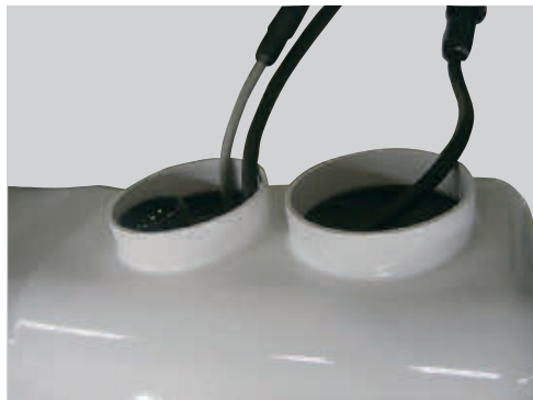
Cables removed when temporarily inserting cover
